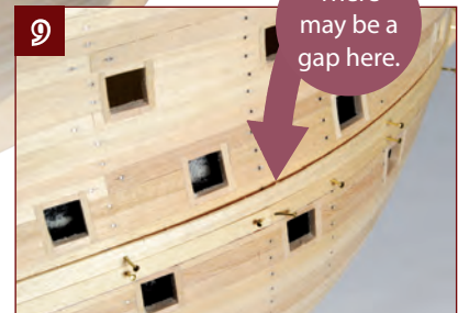
9. Do not be concerned if the top strip does not lie flat against the hull. Any gap where shown will be adjusted later.
